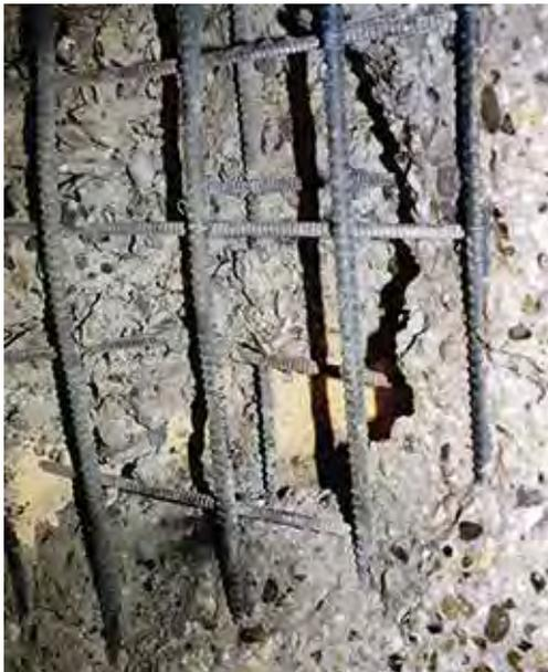
*Concrete silos are often heavily reinforced at the bottom and damage to the reinforcement should be avoided as much as possible.*
