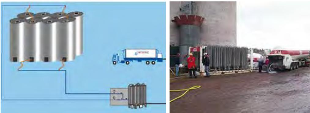
*Inert gas system for silo fire extinguishing (Air Liquide) and photo of a mobile vaporization unit, a gas tank and a tanker (AGA).*
