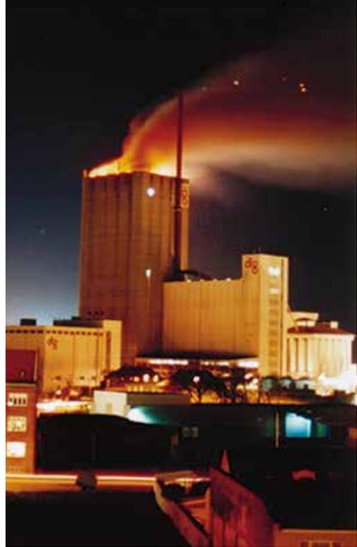
*Fire scenarios that should not need to happen if the appropriate measures are taken, both in preventive work and operational firefighting. The fires in the top of the silos are probably caused by flammable pyrolysis gases that are generated inside silos and which then ignite the top of the silo superstructures.*
