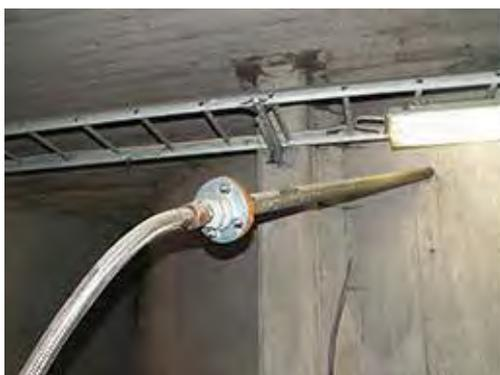
*Examples of temporary gas injections at silo fires by the use of, for example, pipe shaped, perforated lances which are inserted into the material just above the bottom of the silo.*
