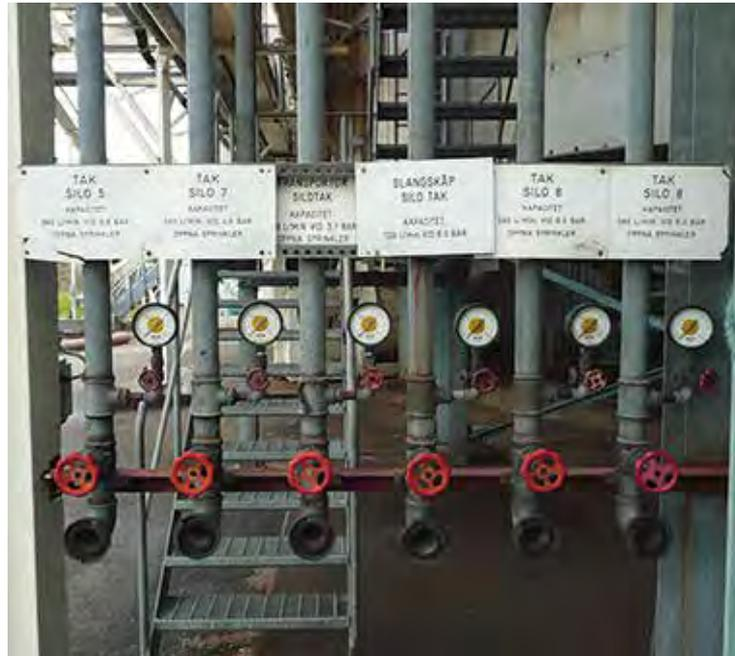
*A fixed riser from ground level facilitates simple and safe application of extinguishing agents into the silo headspace.*
