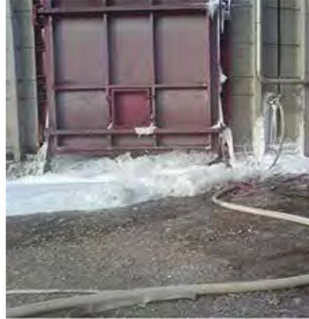
*Application of medium expansion foam onto a peat silo fire, partly through applying the foam via an open hatch (poses a risk of gas explosion in the initial phase) and partly through a hole in the silo wall where a thermal imaging camera has been used to detect hotspots on the inside of the silo wall.*
