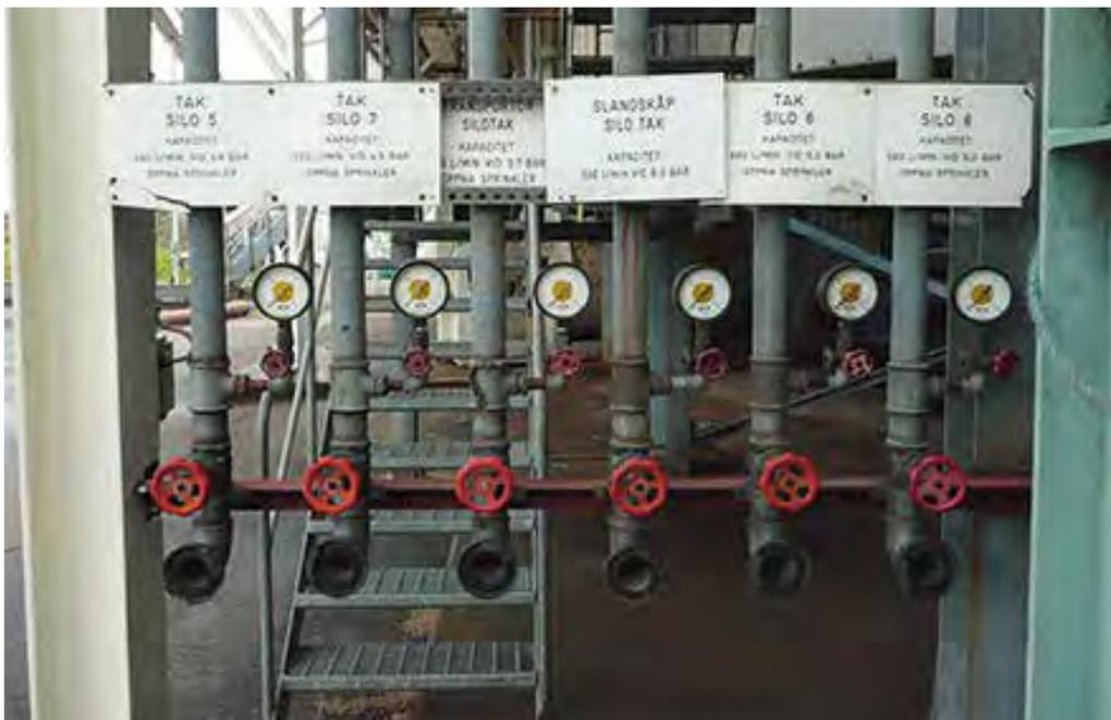
ler system in the silo headspace, which the fire & rescue service can connect to from ground level, such a system could be designed to provide proper function with both water and foam, but also for injection of inert gas if needed.
