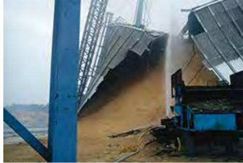
*A silo might tip over if there is an uneven load distribution inside the silo. If pellet material is exposed to water application, it can swell so much that the silo is forced apart.*
