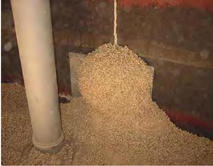
*Because the moist out-door air could flow into the silo, the stored wood pellets swelled and formed a cake at the opening.*
