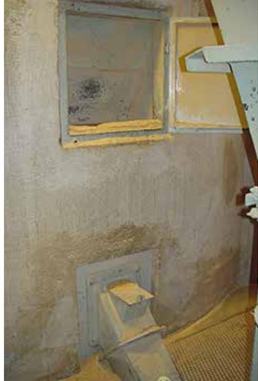
*Examples of openings, conveyor system, ventilation pipes etc., that may need to be sealed, both at the top and bottom of the silo. In older silos made of concrete, there are often openings between the silo cells under the silo roof, which may make it necessary to seal adjacent silo cells as well.*
