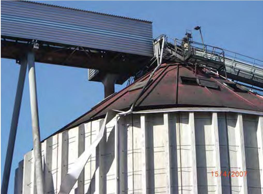
*Example of a dust explosion that lifted the entire silo roof and moved it out of position. The fixed riser to the silo top was also damaged.*
