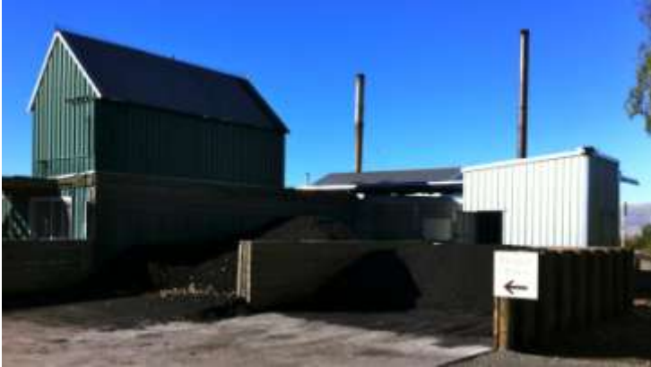
Two coal boilers
