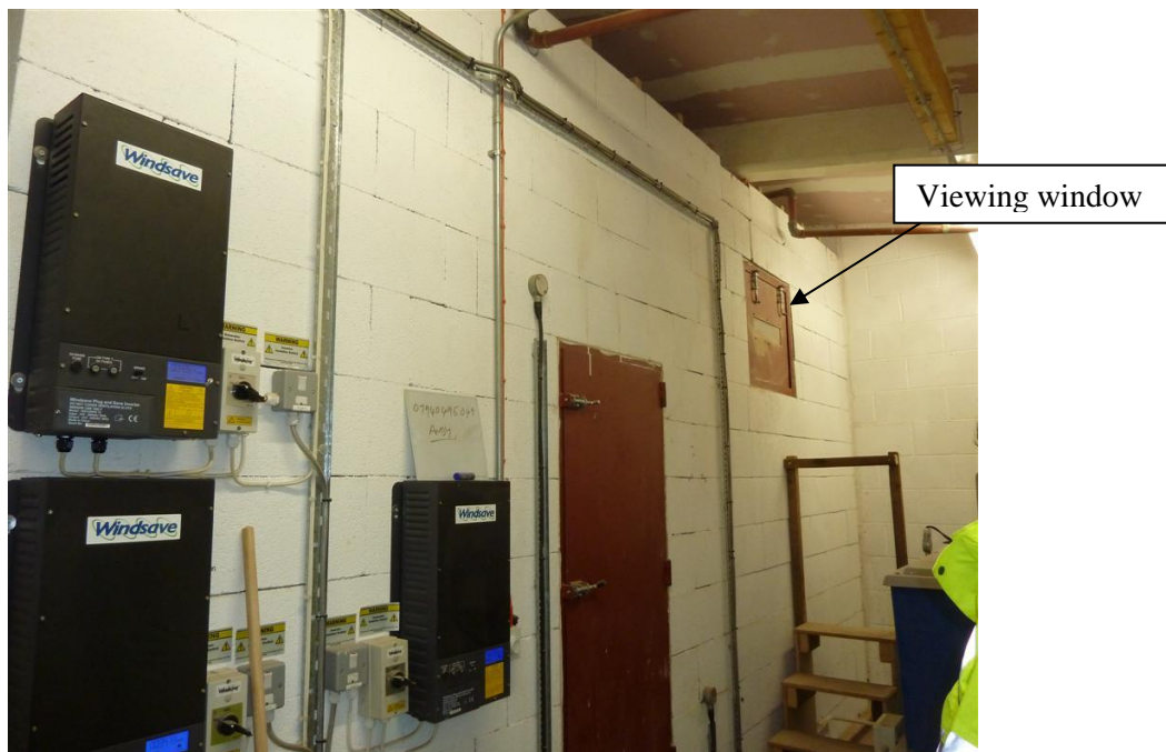
Photograph 2 Site 2 wood pellet store
