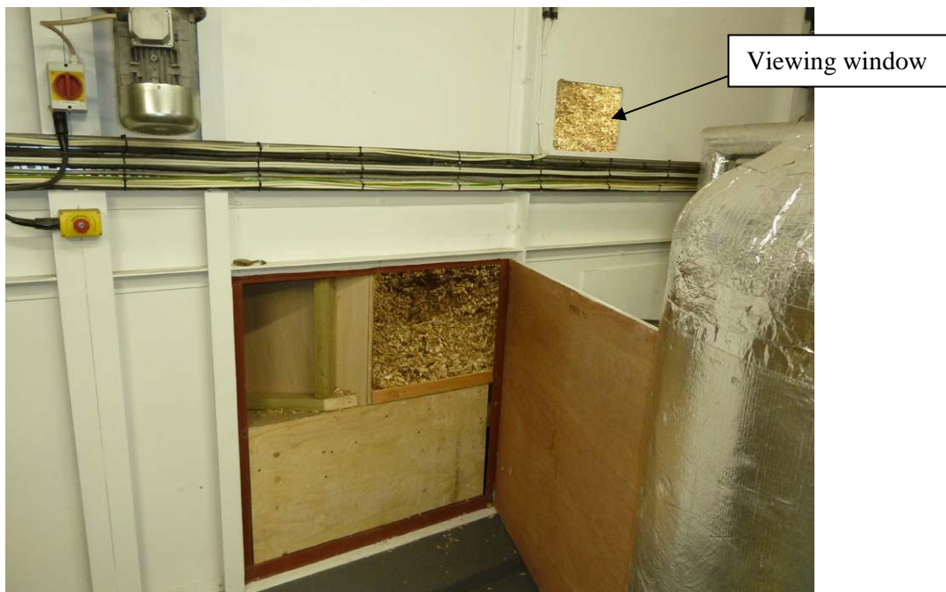
Photograph 5 Site 3 wood chip store access hatch in the boiler room
