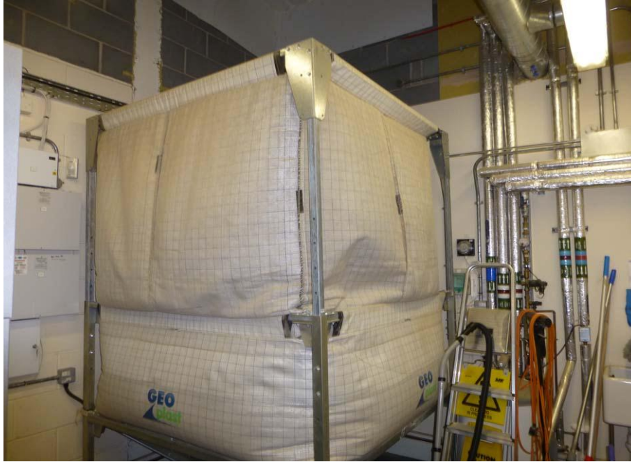
Photograph 9 Site 6 wood pellet storage silo in the boiler room
