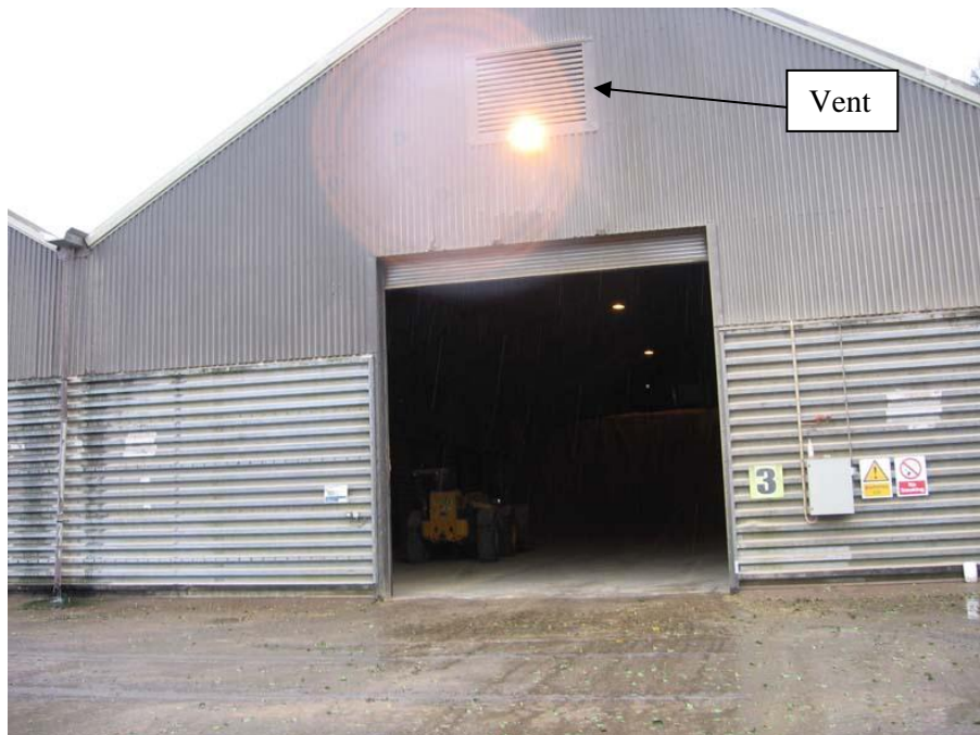
Photograph 10 Site 7 wood pellet storage facility
