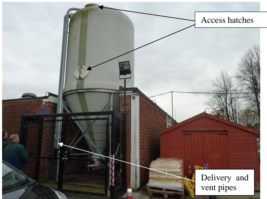
Photograph 1 Site 1 pellet storage silo
