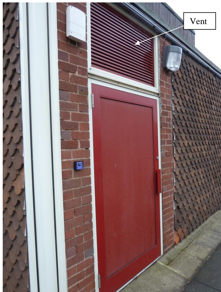
Photograph 7 Site 5 wood pellet store
