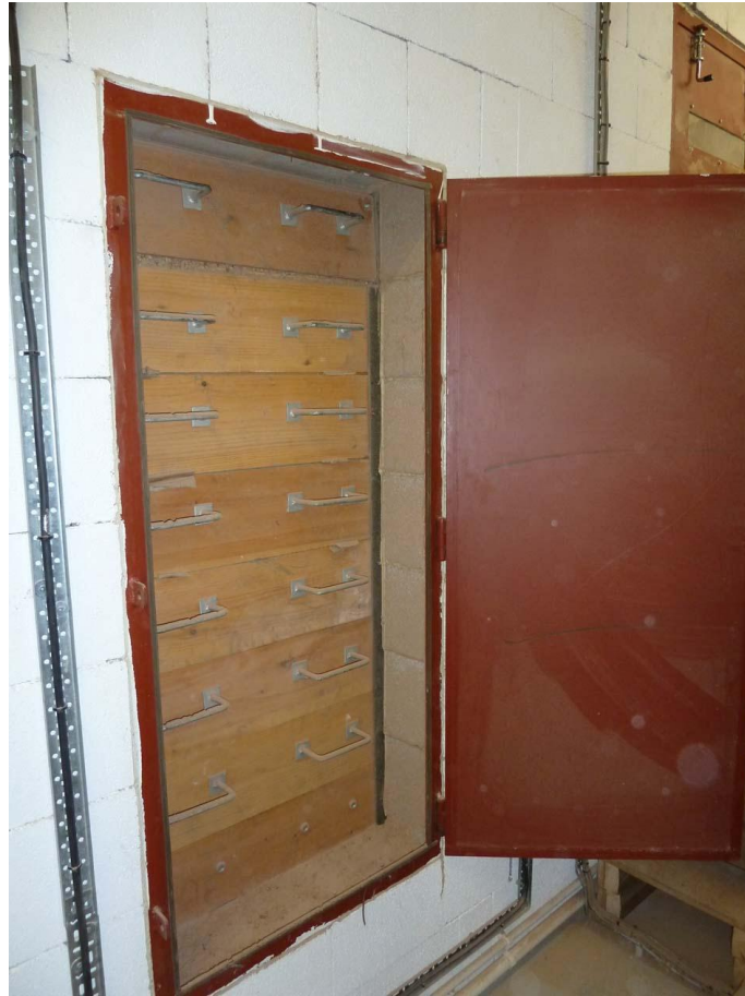
Photograph 3 Site 2 open access door to the pellet store
