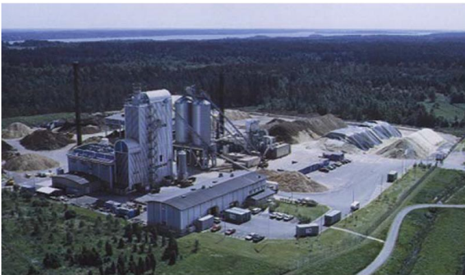
Figure 33: Picture of Värnamo demonstration plant, Sweden [23]
