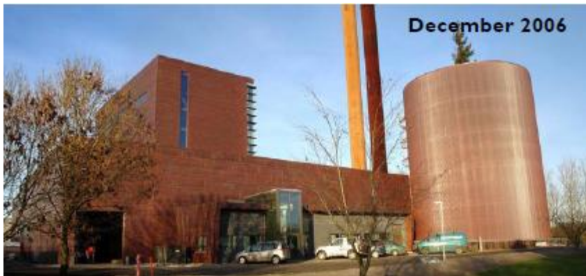
Figure 59: Photo of Skive plant [39]
