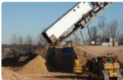
Figure 46: Unloading a semi-trailer at a large scale CHP plant in North America.
