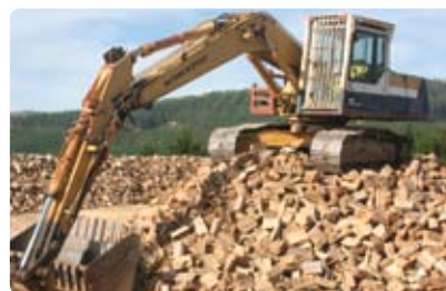
Figure 62: Excavator with a tined bucket, used to both pile for drying, as well as load out firewood.
