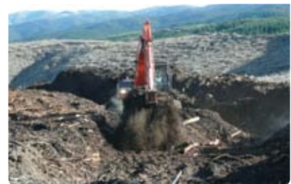
Figure 25: A 20 tonne excavator 'sieving' out biomass that was pushed off the landing during harvesting operations. Here the operator had to work three or four hours to extract 20 tonne of contaminated wood fuel.
