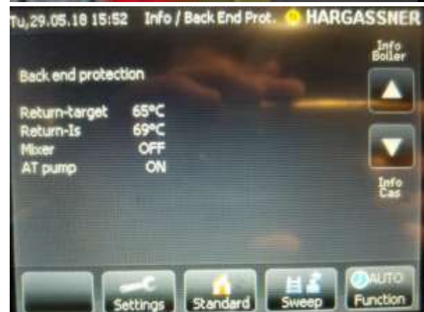
Fig. 9 and 10: The ex-factory back-end protection, and screen showing the set point for the min return temp
