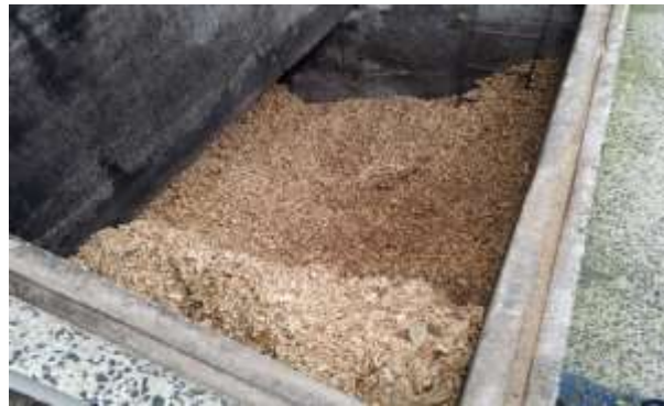
Fig. 27: fuel store, with a volume-limiting back wall – not important when it was coal
