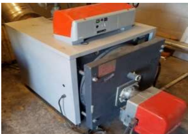
Fig. 20 and 21: An 88kW ETA Hack wood boiler and a 93kW diesel back-up
