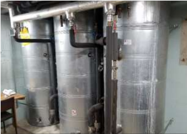
Fig. 11 and 12: The 2 x 1500 litre insulated accumulator tanks (left) and 3 x 500 li calorifier tanks
