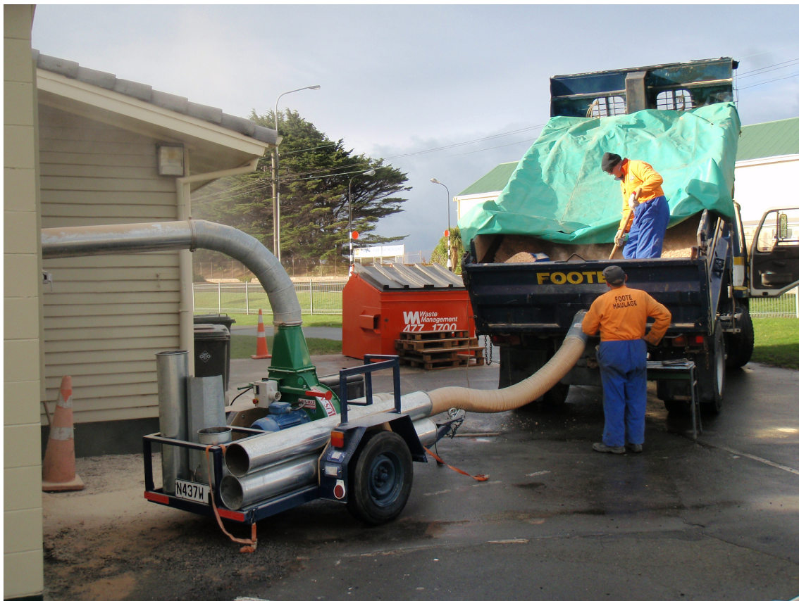
Figure 1 Wood chip blowing from the truck to the wood chip bunker
