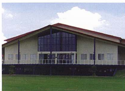
The new events centre.
