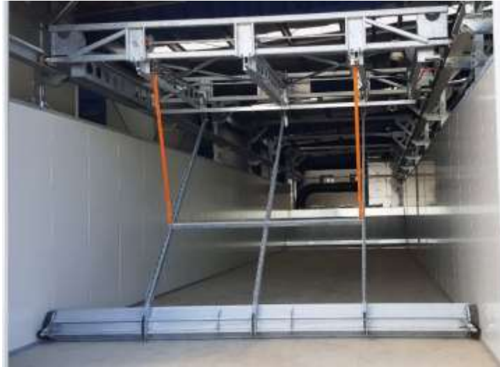
A Toploader in a 450m 3 fuel bay feeding a wood boiler at a glasshouse near Sydney
