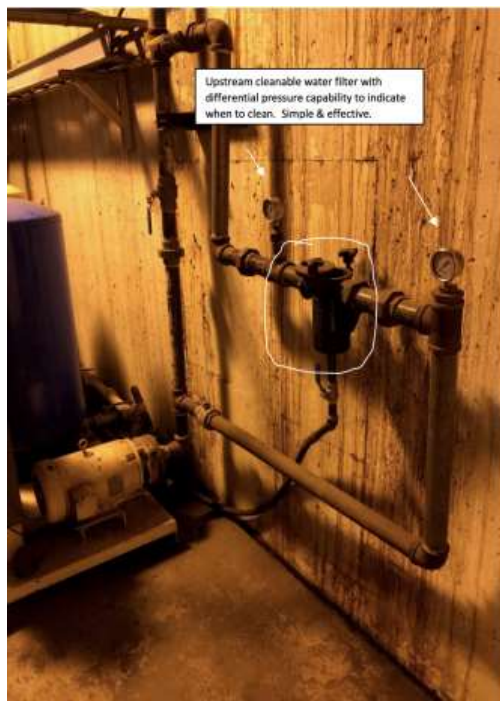
Upstream cleanable water filter with differential pressure capability to indicate when to clean. Simple and effective.
