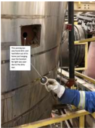
This sensing eye was found dirty and had fallen out of its home, just hanging over the handrail. No light was seen because of the dirty eye.
