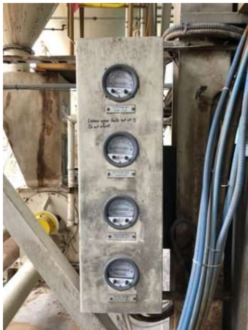
An example of a photohelic that has had the alarm threshold increased above 5"WC.
