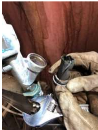
Water supply line to deluge nozzle in-line strainer requires frequent cleaning, otherwise water flow could be reduced or blocked. Note: this strainer was leaking due to damaged threads.
