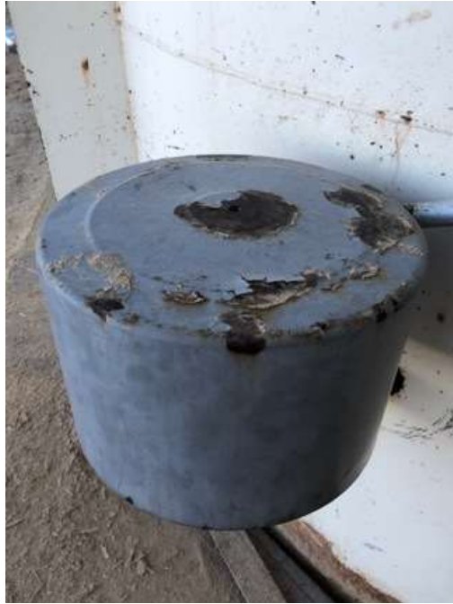
Missing fastening nut results in a poor seal.
