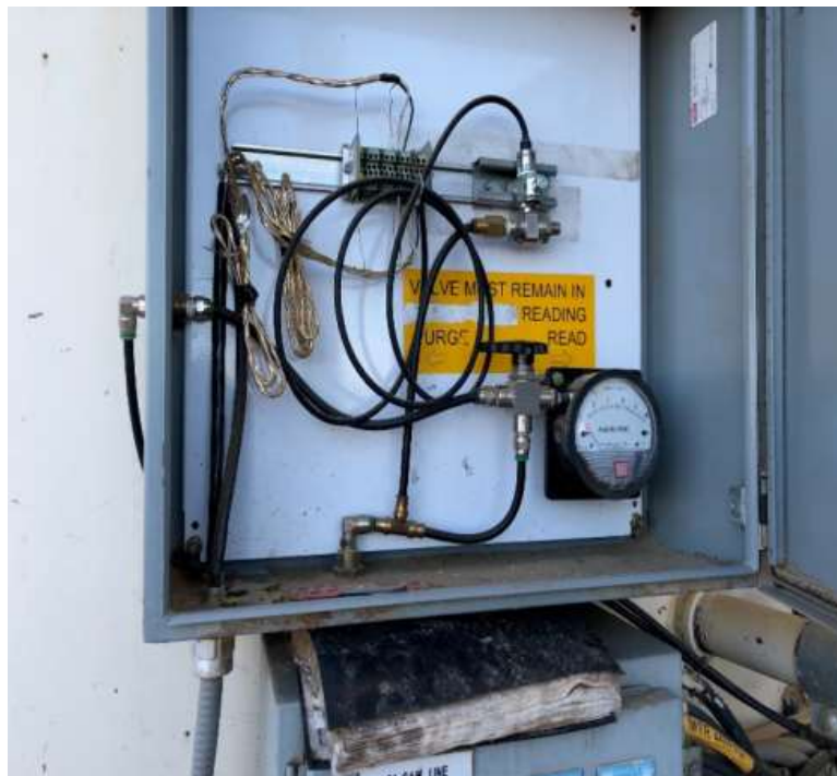
Example of poor installation.
